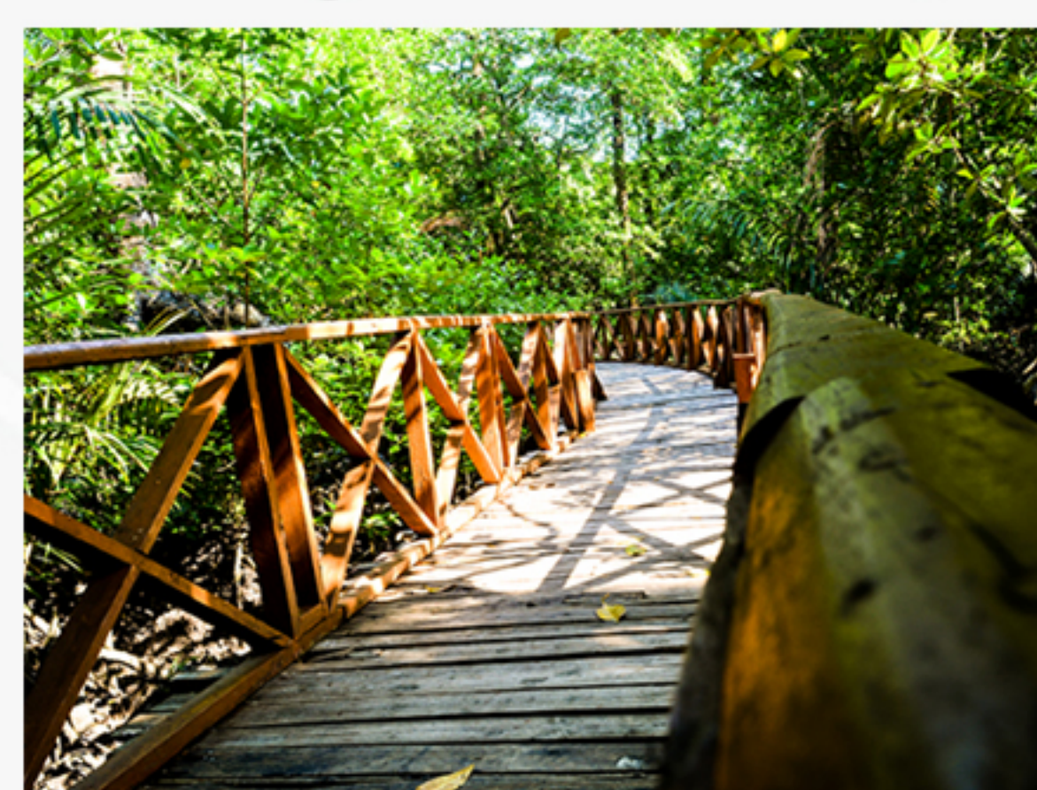
Dhani Nallah Mangrove Walkway
